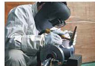
MIG Welding Repair
