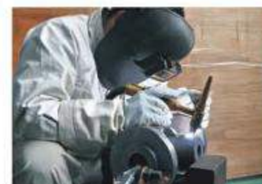
MIG Welding Repair
